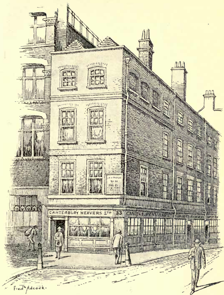
OLD HOUSES—MILK STREET, CHEAPSIDE RECENTLY DEMOLISHED
